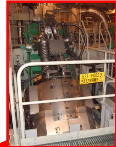
主蒸気隔離弁(8台)
